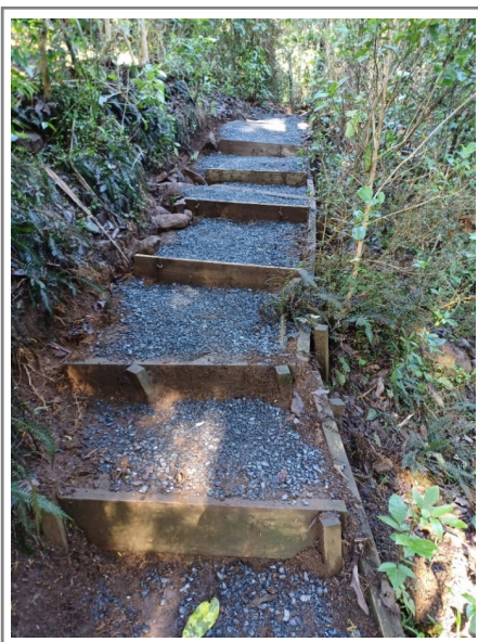
These steps have been upgraded
