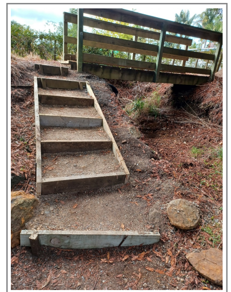
These steps have been tidied up
